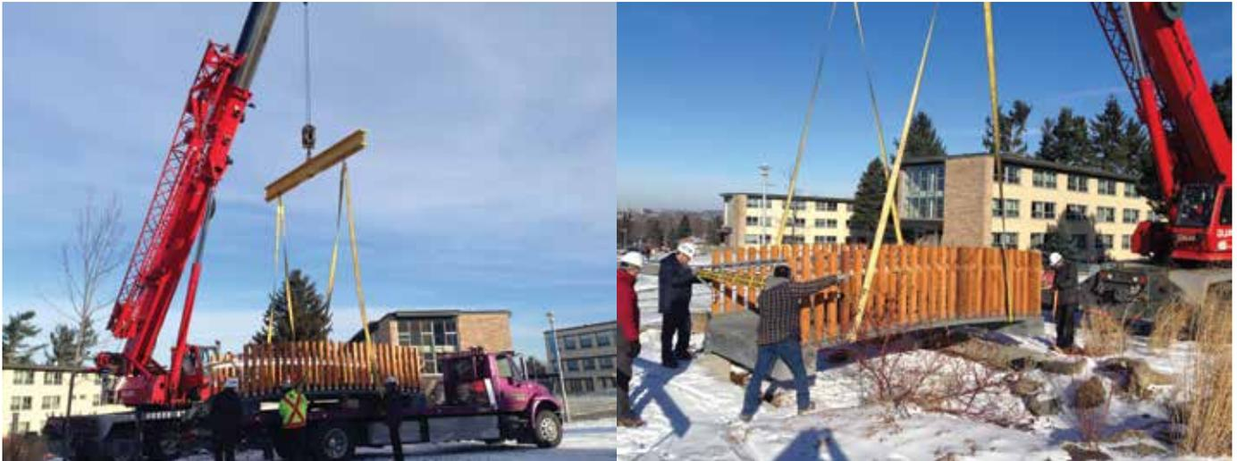
Fig. 5: The completed footbridges were transported on a flatbed truck and installed with a truck-mounted crane
