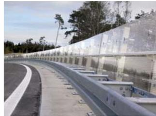
Fragment retention feature controls falling debris if struck by an errant vehicle
