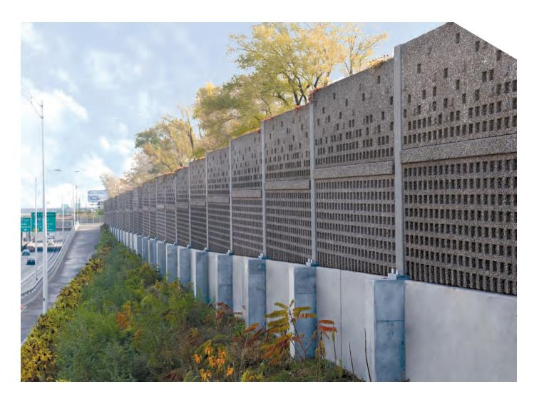
SOUND-ABSORPTIVE WALLS MADE FROM A UNIQUE COMBINATION OF RECYCLED RUBBER TIRES AND STRUCTURAL CONCRETE
