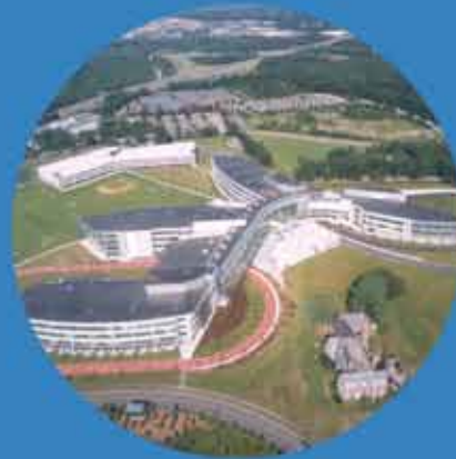
Reebok World Headquarters, Canton, MA
